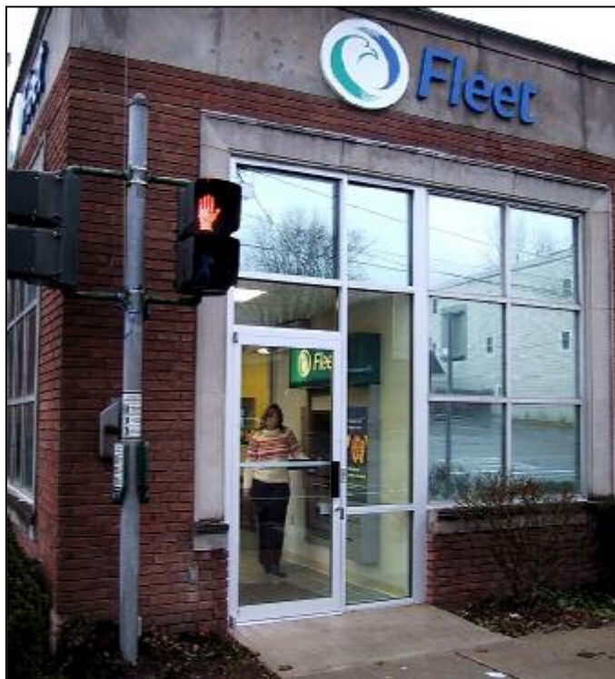
Below, Sales Assoc. Venetia Perkins of Fleet Bank shows off their new handicapped-accessible ATM entrance & vestibule on Main St.
